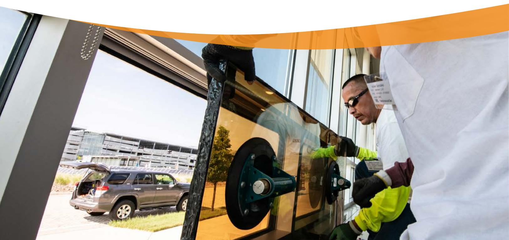
Glazers install one of five quantum dot windows from UbiQD at the NREL Cafe. The windows will remain installed for one year as NREL and UBIQD collect data. Quantum dot laminated glass absorbs sunlight and the glow from quantum dots is trapped in glass by internal reflection and guided to the solar cells at edges to generate electricity. *Dennis Schroeder, NREL 64976*
